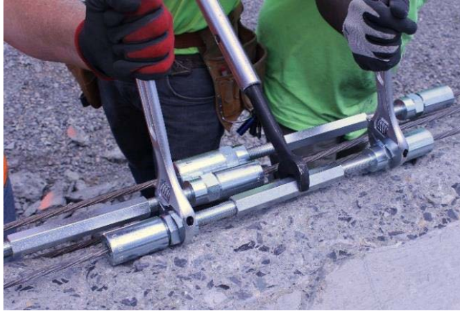
Figure 1. Installation of Splice Chucks
