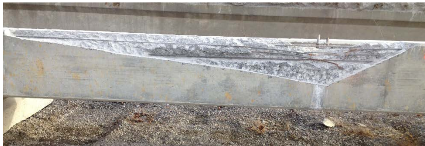
Figure 25. Beam D after Chipping and Saw Cutting
