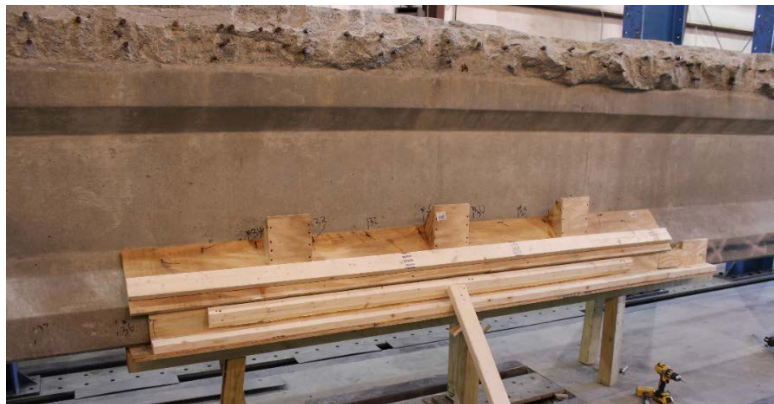
Figure 16. Formwork for Concrete Placement
