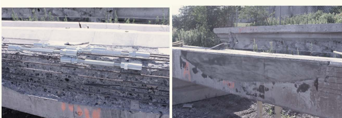
Figure 21. Completed Installation of the Strand Splices and Beam after Form Removal
