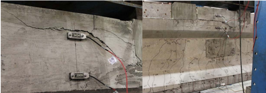
Figure 56. Test 4 Flexural Compression Failure in the Deck (left) and Cracking Pattern in Beam Below Load Point (right)
