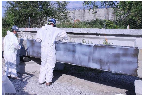
Figure 22. Spreading Putty over Area of Beam to be Repaired
