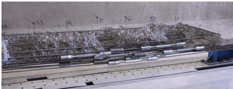
Figure 15. Completed Installation of Strand Splices
