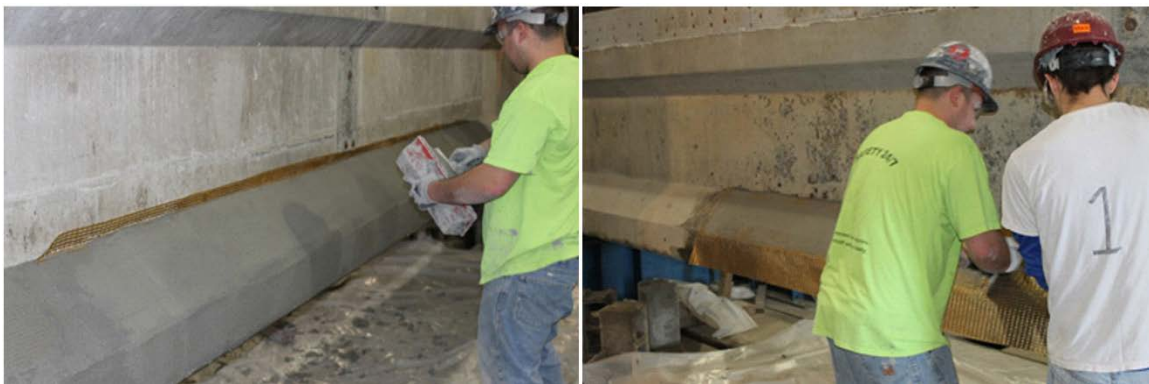
Figure 27. Trowling Mortar over a Layer of Mesh and Pressing Mesh into Layer of Mortar
